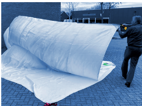
Make sure the blanket is high enough to prevent it from snagging and thereby damaging it
